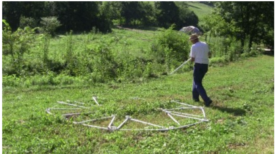
Attach 20 Struts and 10 Hubs to make 10 Blue Triangles
